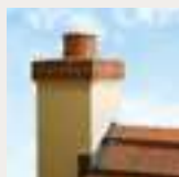
Brick or Stone Chimney (Class 1)
