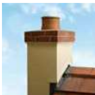
Brick or Stone Chimney (Class 1)
